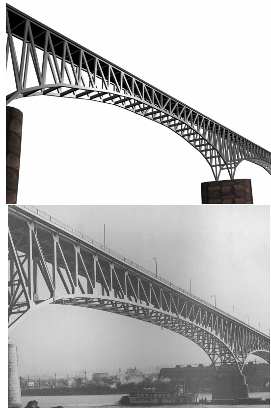
Figure 1: A cantilever bridge generated by our software, compared with the Homestead bridge in Pittsburgh, Pennsylvania.
