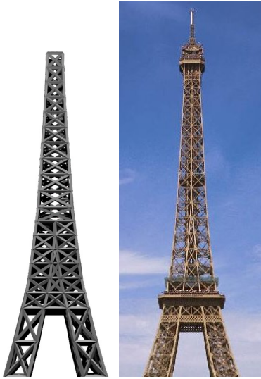
Figure 9: Our trusswork tower, compared with a detail of the Eiffel Tower. Because they are ornamental and not structural, the observation decks are not included in our tower.
